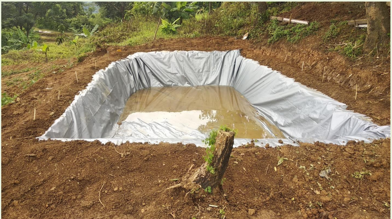
Low cost rain water harvesting structure 'Jalkund'
