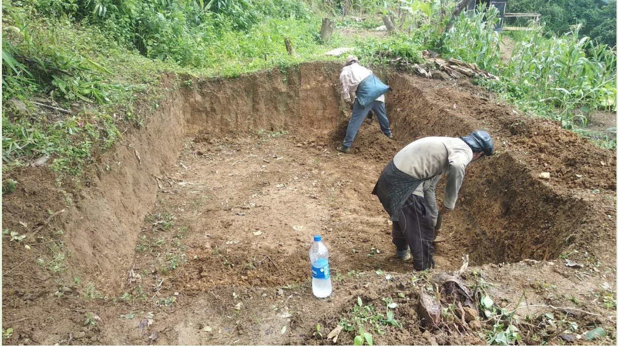
Excavation of farm pond inconvergence with MNREGS
