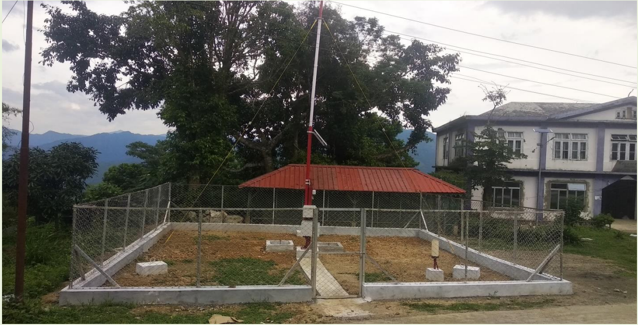
Automatic Weather Station at Hnahthial
